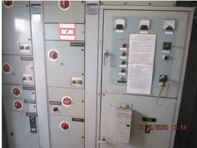
Emergency Switch Board room
