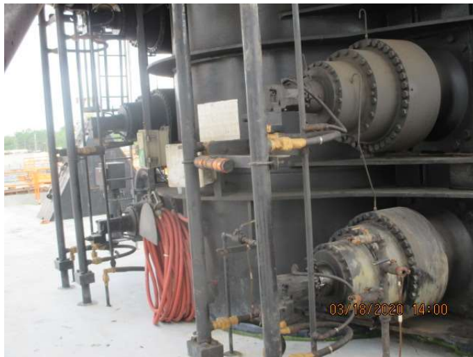
Stbd Fwd Jacking system
