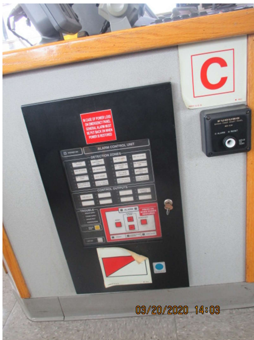
Fire Alarm panel on bridge
