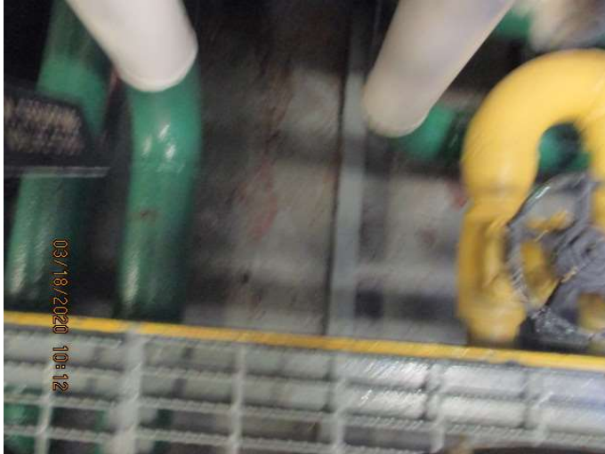
Engine room bilges
