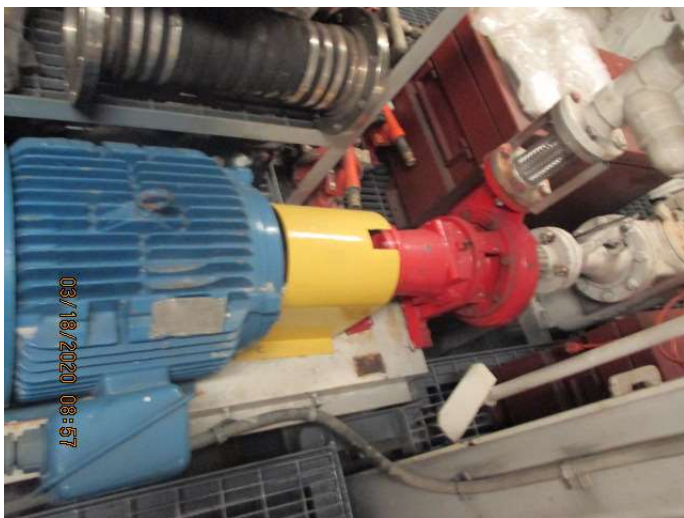
Fire Pump in Stbd Engine room
