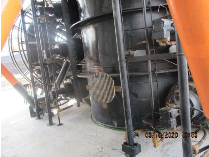
Aft Jack house front view
