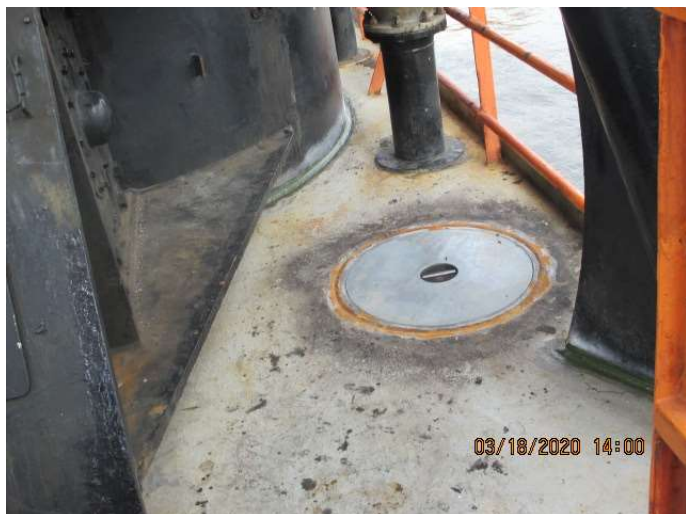
New manhole cover
