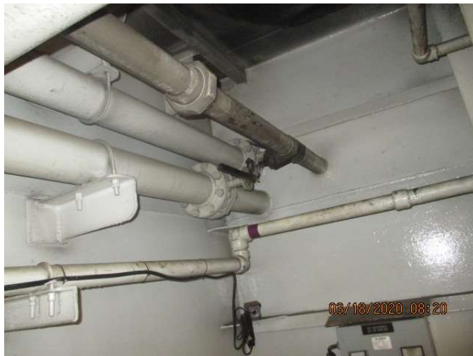
Pipe Penetration inside engine room
