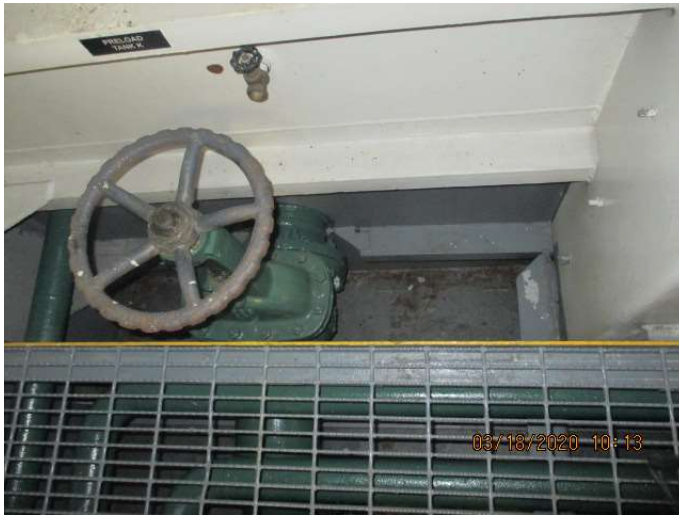
Preload tank valve
