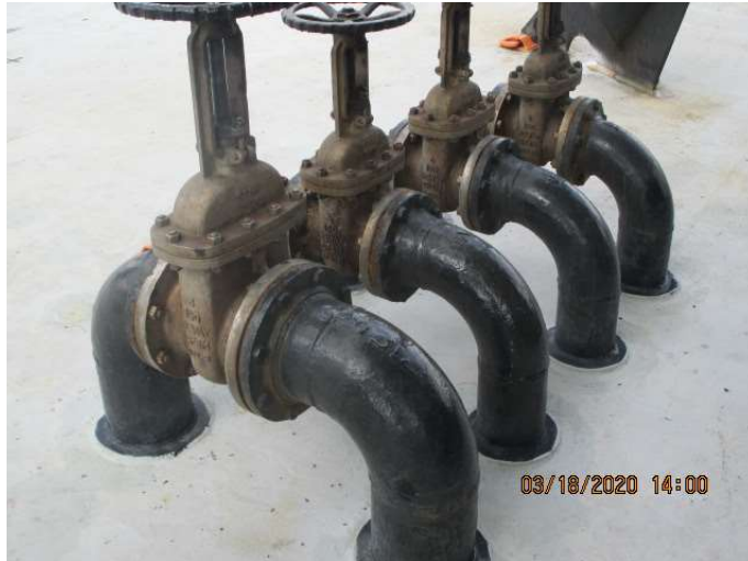
Preload Tank Valve on deck
