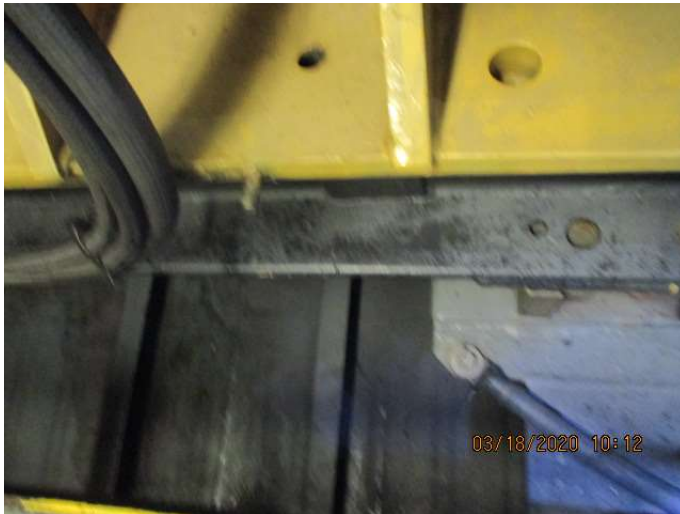
Engine room bilges
