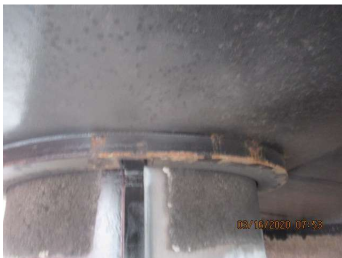
Stbd fwd jack house lower hull connection
