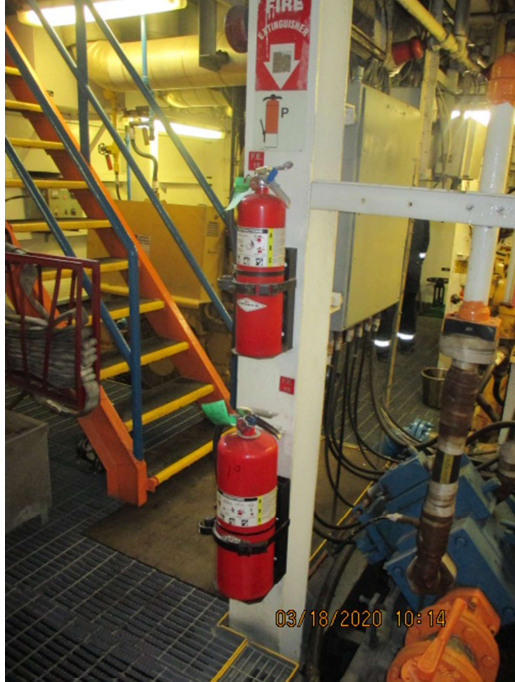
Port engine room
