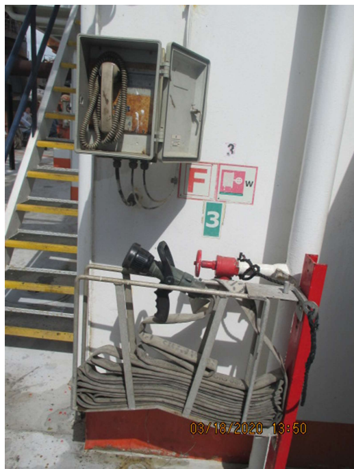
Fire Hydrant on aft Main deck behind accommodation
