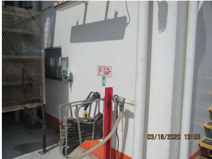
Fire station on main deck aft stbd
