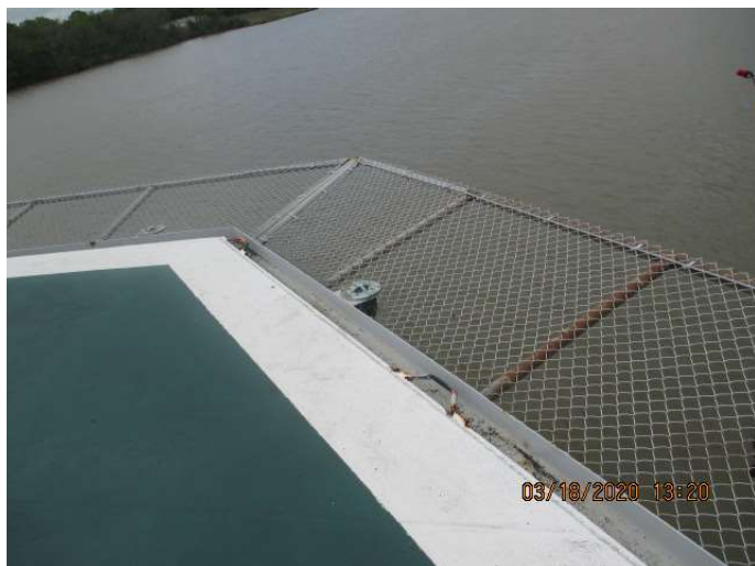
Safety Net on heli deck
