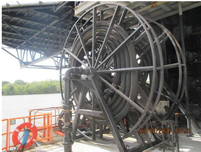
Raw water hose reel on stbd aft main deck
