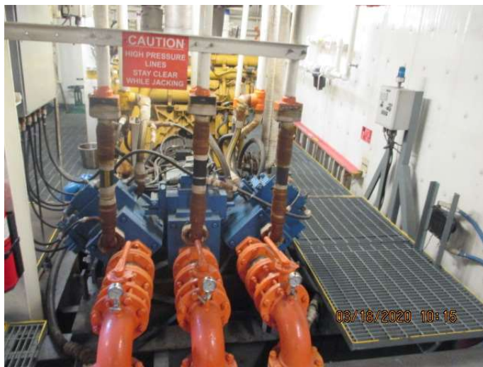
Jacking Hydraulic pump on Inboard Main engine
