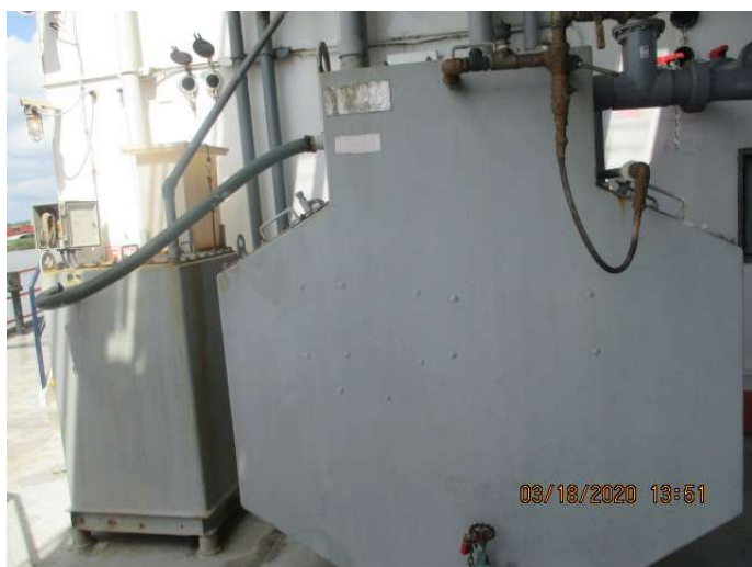
Sewage treatment plant Aft Port side on main deck
