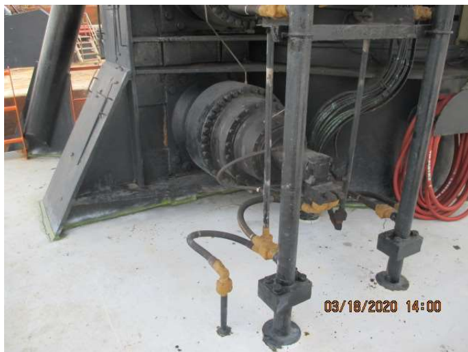
Jacking system hydraulic connection
