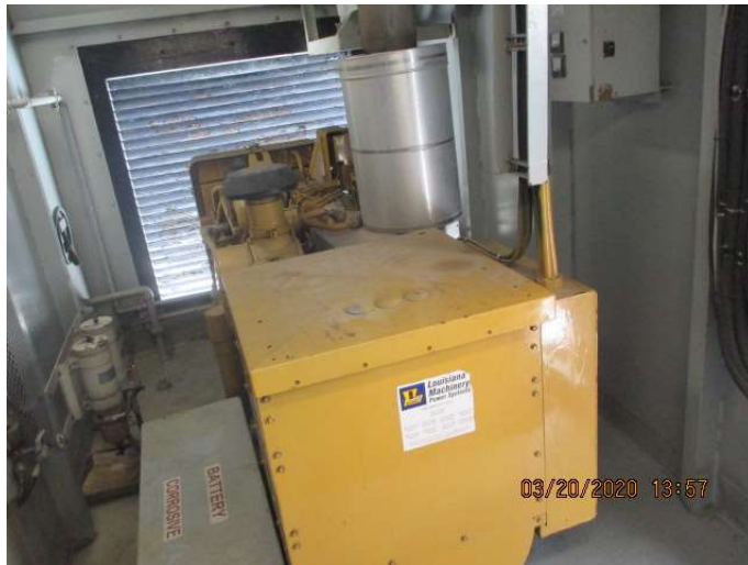
Emergency generator room
