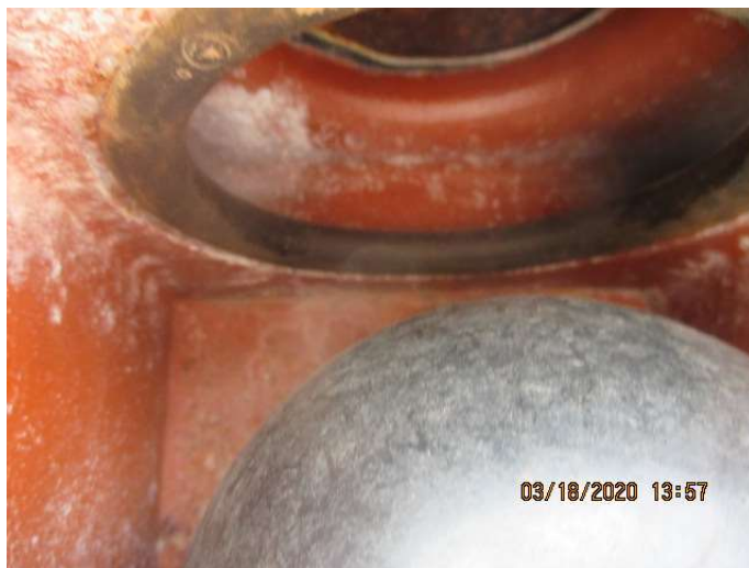
Air vent Inside with float ball and gasket
