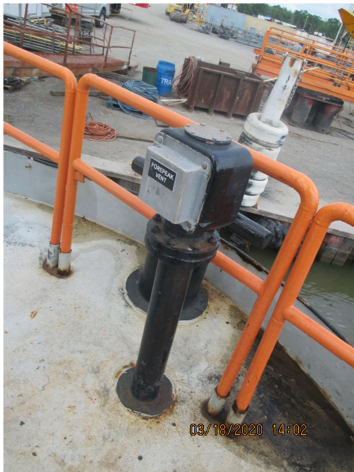
Air vent pipe stbd forward
