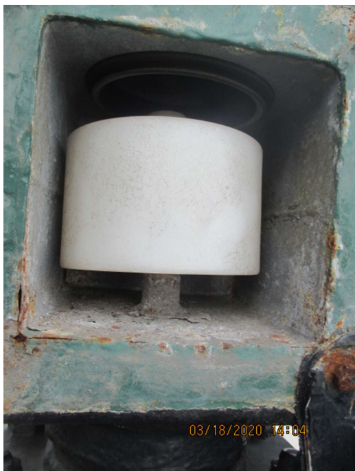
Air vent pipe
