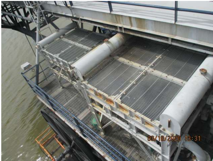
Stbd side Radiator
