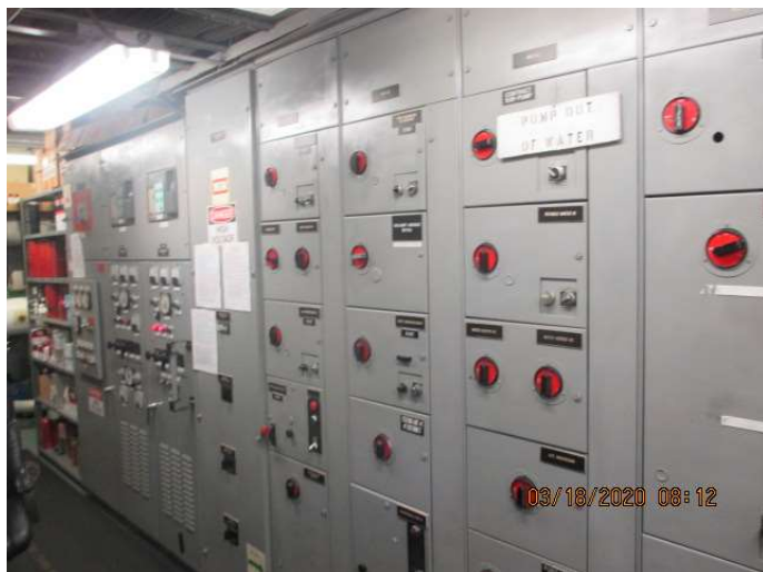
Engine Control Room Switch board
