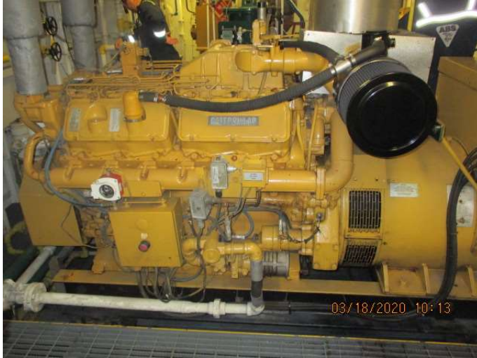
Aux engine Port side Engine room
