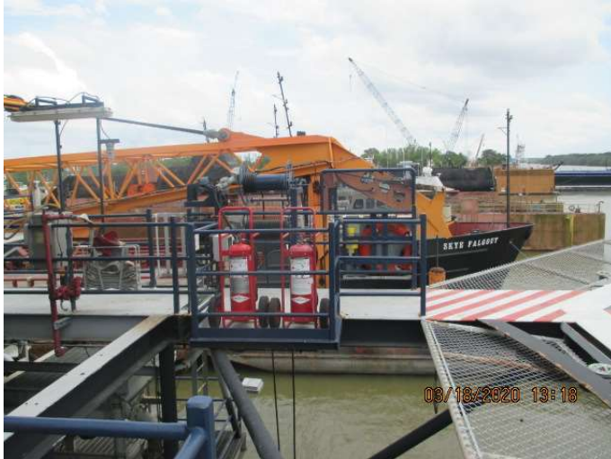
Trolley Fire extinguisher for heli deck
