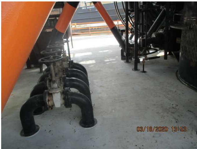
Aft preload tank valve manifold
