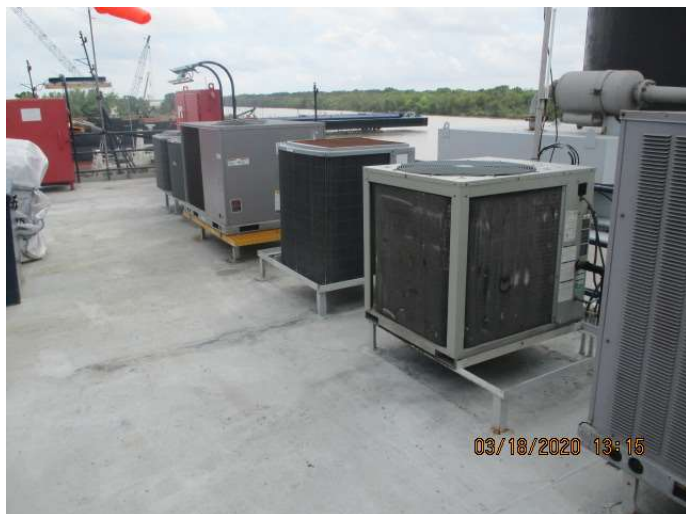
Bridge aft View
