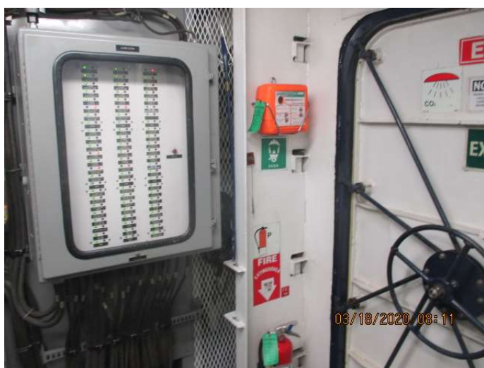
ECR Port side alarm panel
