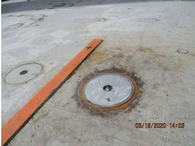
New manhole cover
