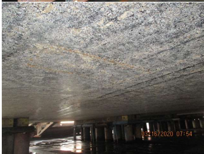
Bottom Hull View
